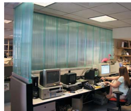
The Gallina 344 product is another example of polycarbonate used for security, privacy and noise reduction purposes.
